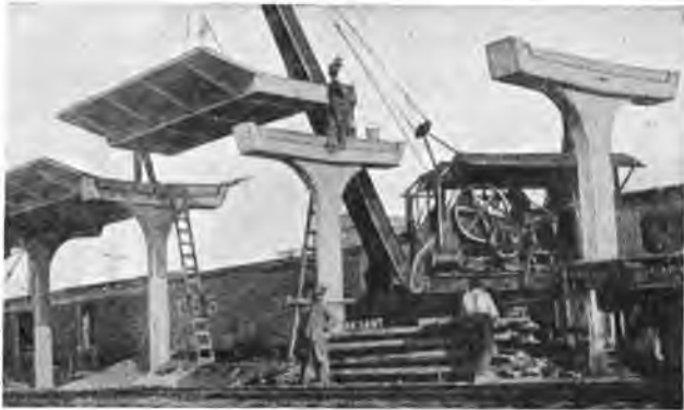
Fig. 161a. Placing Roof Slabs.
